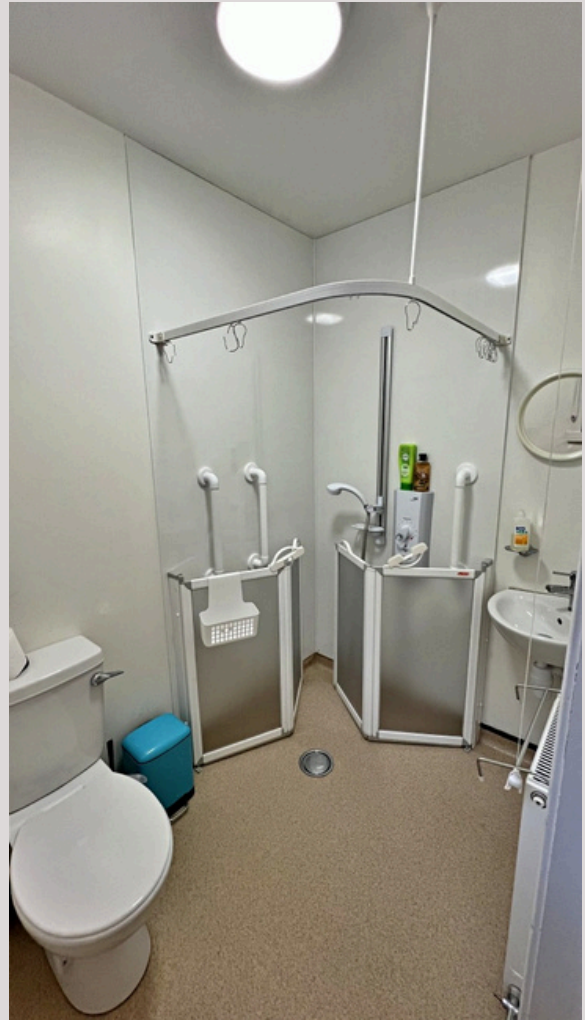
Shower Room - 1.92m x 1.38m
